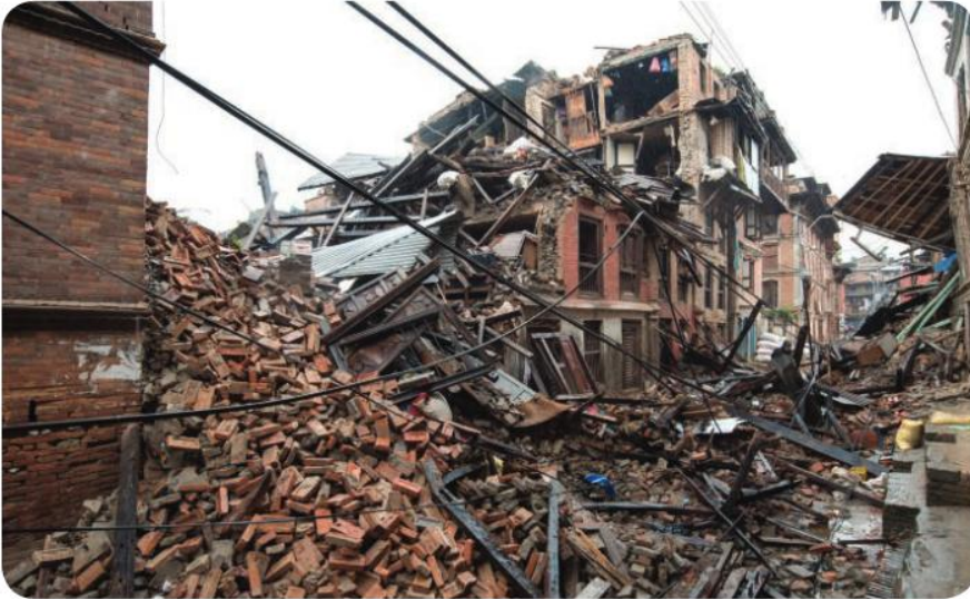
◀ This photograph was taken after the 2015 earthquake in Nepal, which had a magnitude of 8.1
